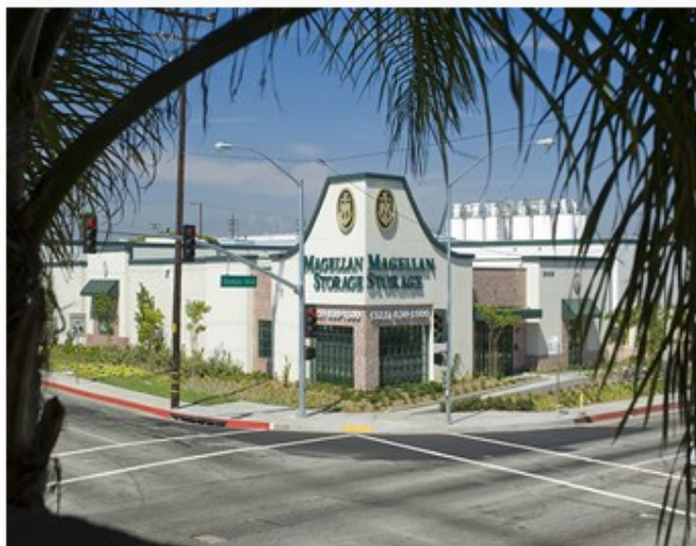
Magellan Storage—Commerce, 5415 E. Olympic Blvd., Commerce, Calif.
